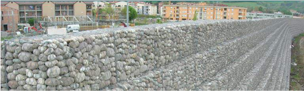
Figure 10E.8: Gabion walling noise barrier
