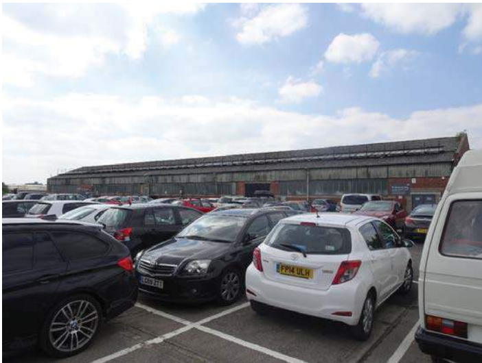
Plate 5. B37 brick/ corrugated steel buildings
