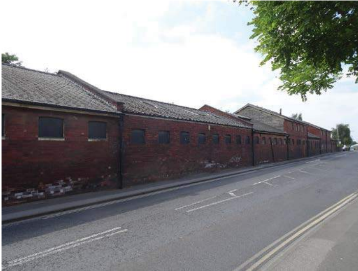
Plate 4. B36 old brick-built buildings
