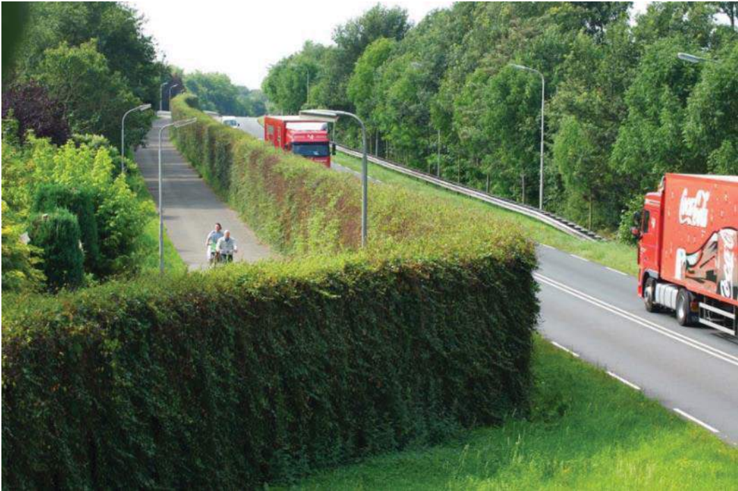
Figure 10E.9: Planted noise barrier
