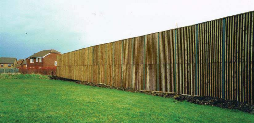
Figure 10E.7: Timber fence noise barrier
