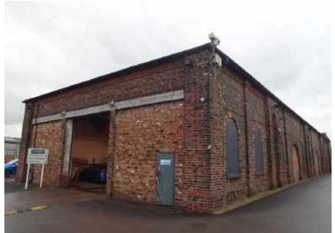
Fig.250 Albion Iron Foundry shop - main building - east facade
