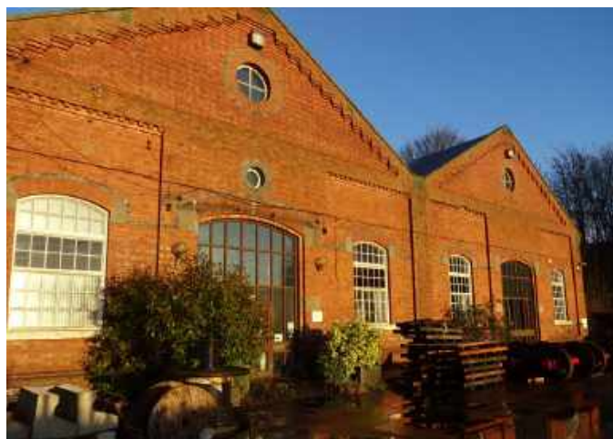
Fig.268 Carriage works stores and office, also known as Alliance House
