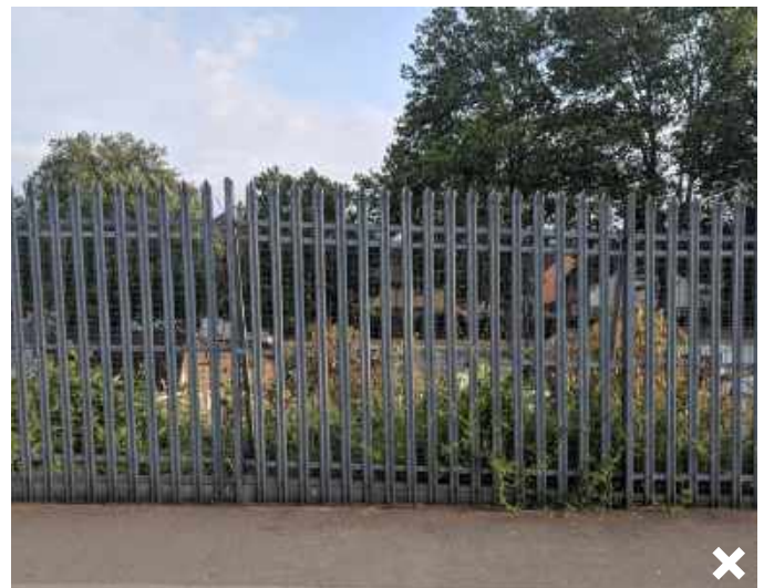
Fig.380 Palisade fencing is not a preferred fencing type. Raw steel/metal finishes are not appropriate
