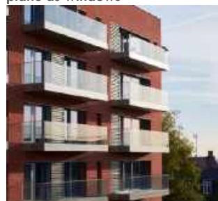
Glass balustrade to projecting balconies ✗
