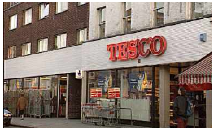
Fig.354 Shopfront fascia dominates building
