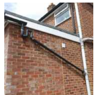
Fig.312 Ill-considered downpipes
