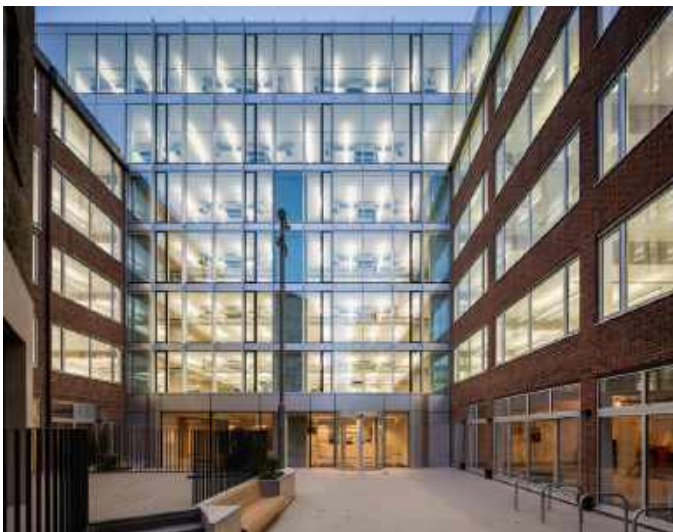
Fig.422 Fully glazed wall, Sutton Yard, Islington London
