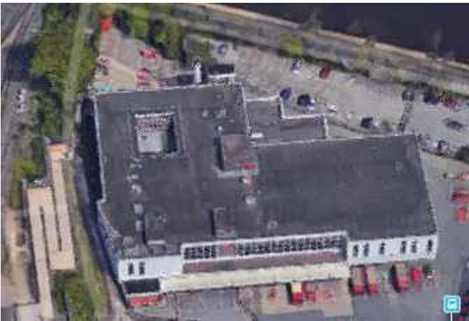
Fig.288 Large flat roof to Post Office ❌
