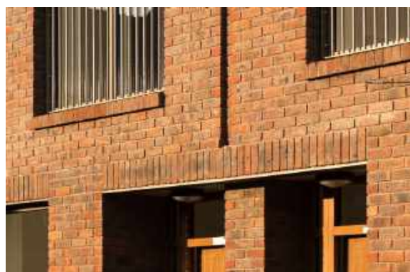
Example of cill and head details, and brick recesses used to articulate brick facades
