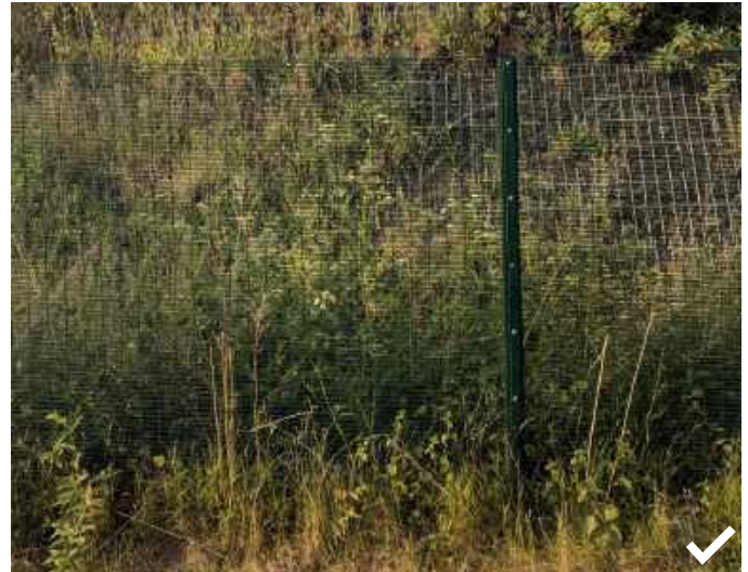
Fig.379 Green mesh blends into landscape. Fence to railway, Millwall
