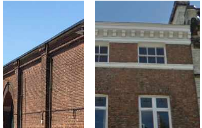
Fig.307 Examples of the many different existing eaves details in York
