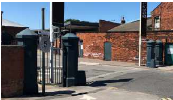
4 Gate Piers (Grade II listed)
