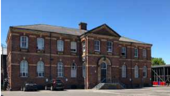
1 Former Goods Station (Grade II listed)
