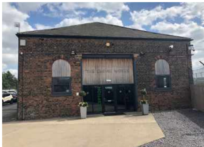
Fig.254 'Engine Shed' north facade
