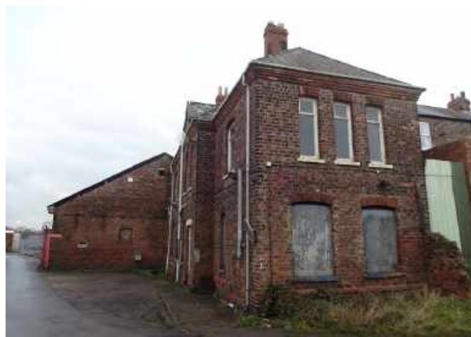
Fig.257 East frontage of Smith's Shop Office
