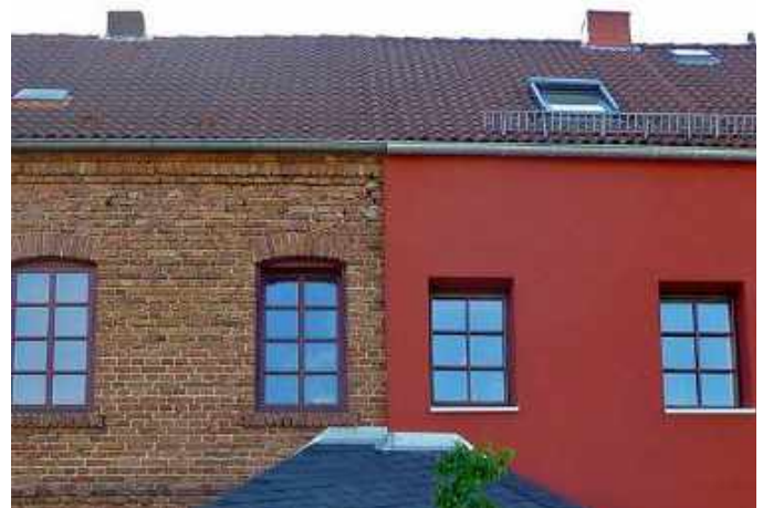
Fig.243 Exterior insulation covering brick details on historic building in Germany
