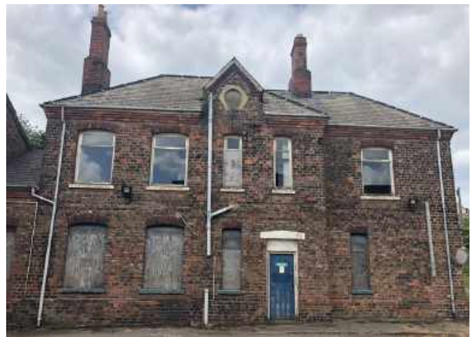
4 Smith's Shop Office
