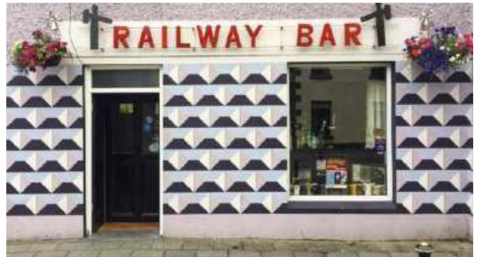
Fig.358 Individual contemporary shopfront design encouraged ✓
