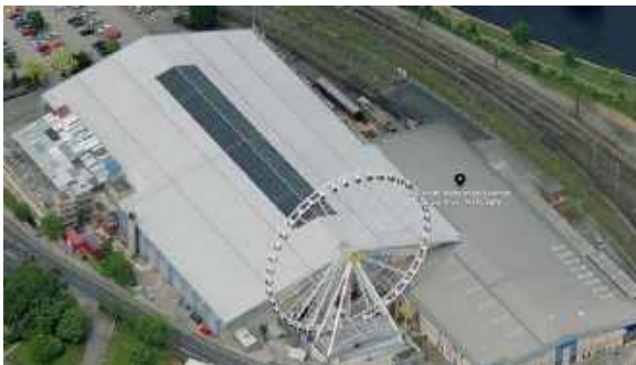
2 York North Engine Shed (non-designated)
