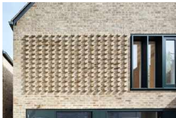
Example of modern relief pattern to enrich brick facades
