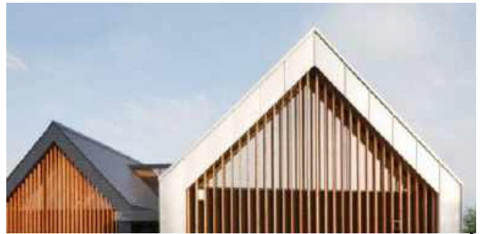
Fig.314 Contemporary modelled verges
