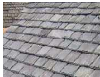
Fig.297 Lake District slates
