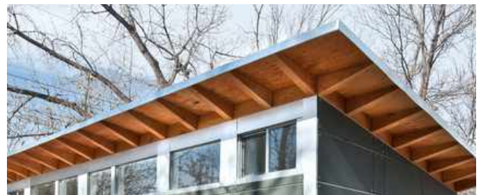
Fig.308 Example of a contemporary eaves detail
