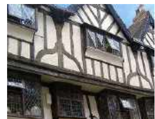
A historic jettied floor in York
