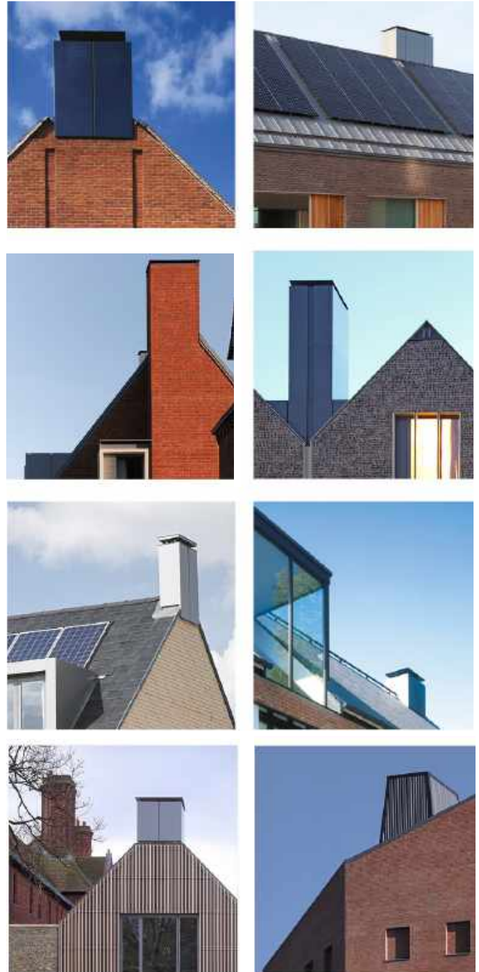
Fig.319 Examples of contemporary chimneys
