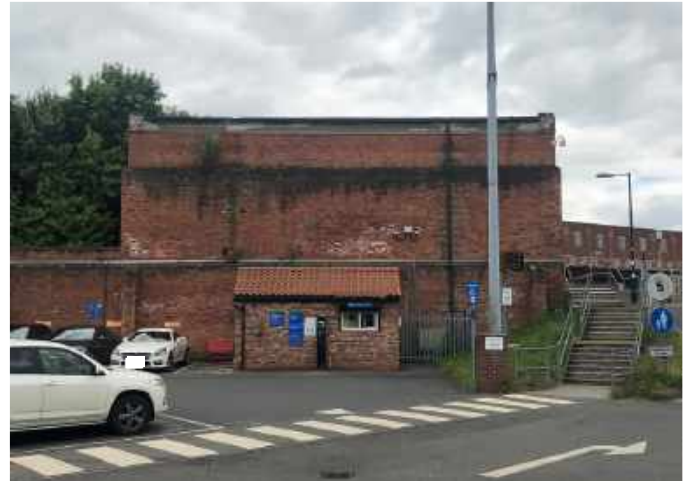
Fig.265 Generator building seen from the west
