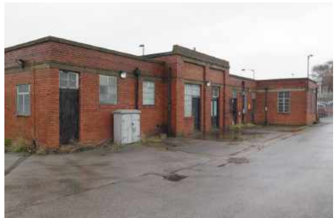
Fig.259 South elevation of 1930s Leeman Road building
