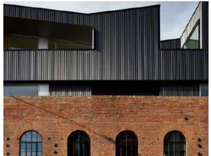
Fig.423 Metal sheeting, Shoreham Street, Sheffield
