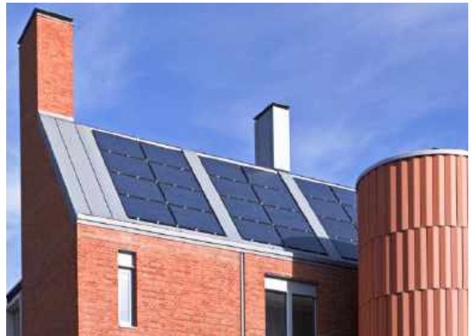
Fig.329 Example of solar roof panels integrated into the roofscape, flush with the roof covering ✓
