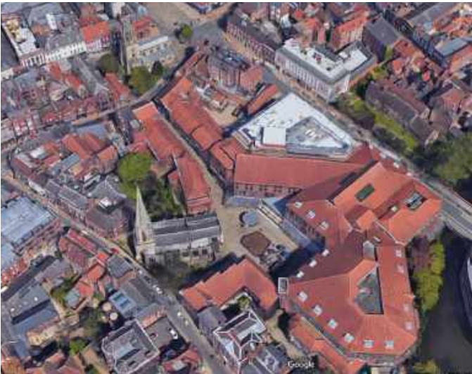
Fig.287 Large scale clay tiled roof to Coppergate shopping Centre ❌
