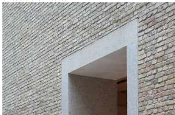
Example of a contrasting masonry material used to frame openings in brick walling
