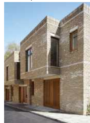
Fig.344 Example of contemporary jettied floors
