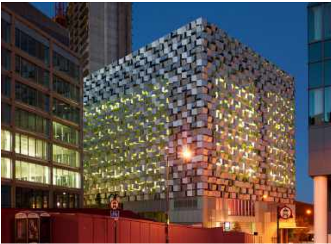
Fig.427 Carpark structure, Charles Street, Sheffield
