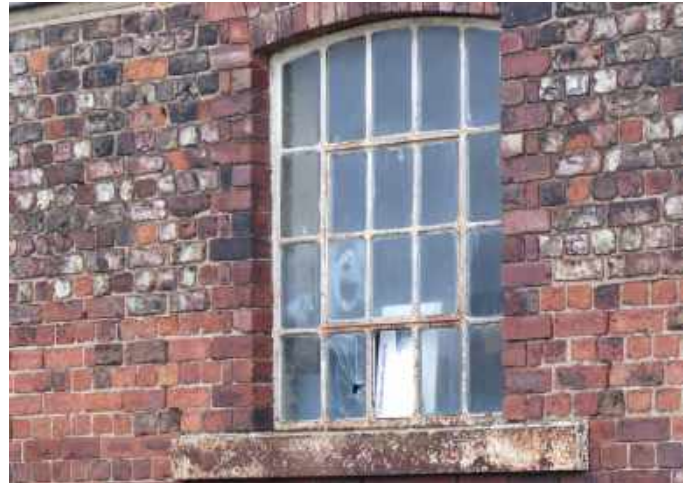
Fig.244 Existing iron window could be retained and repaired
