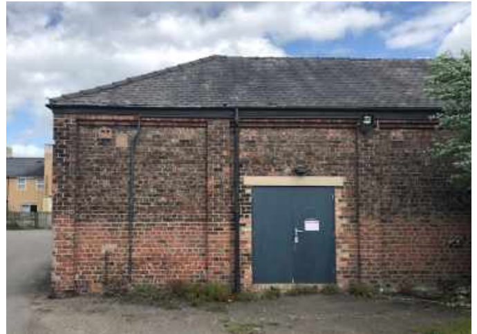
Fig.240 Existing railway shed in the Albion Foundry area
