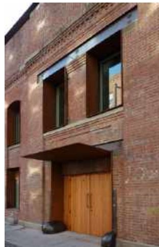
Fig.235 New windows and entrance at the Eberhard Faber Pencil Factory, Brooklyn
