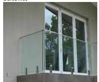
Glass balustrade to a projecting balcony ✗
