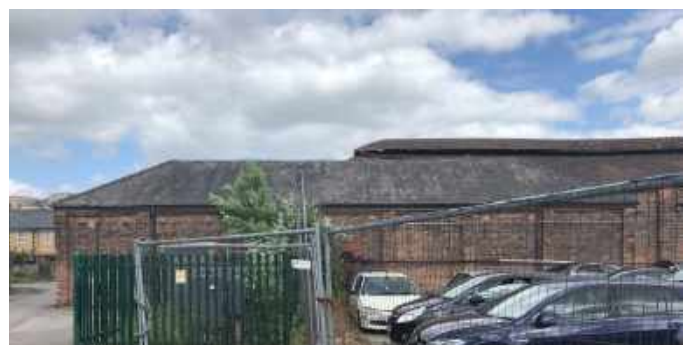
Fig.252 Albion Iron Foundry shop - parallel brick shed - west facade
