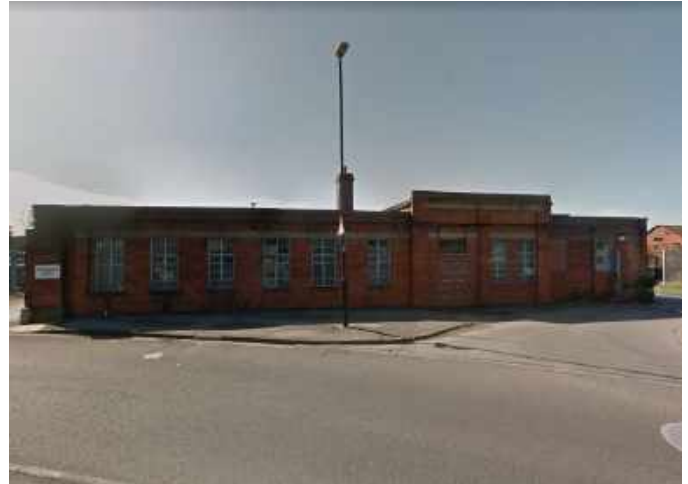
Fig.258 1930s building seen from Leeman Road
