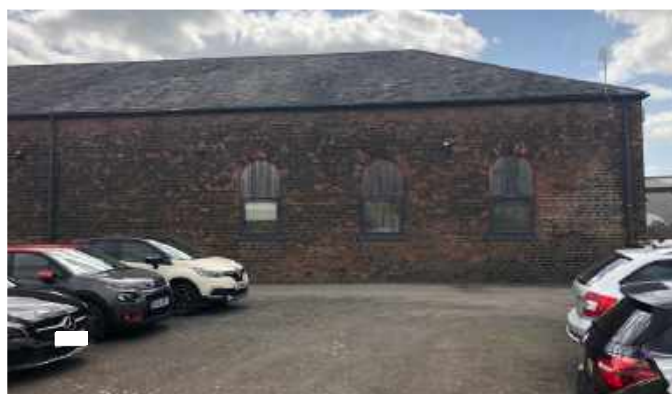
Fig.255 'Engine Shed' north facade east facade
