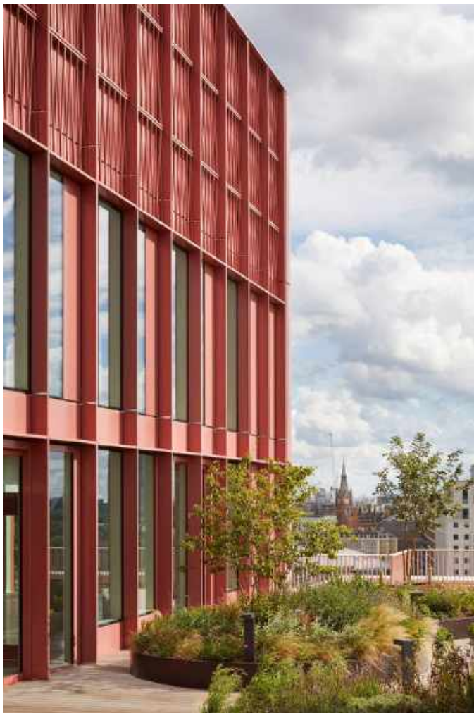
Fig.411 R7 Kings Cross office building, London Contemporary commercial buildings
