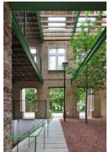
Fig.236 Industrial space re-used, Melle, Belgium, part open space, part care home
