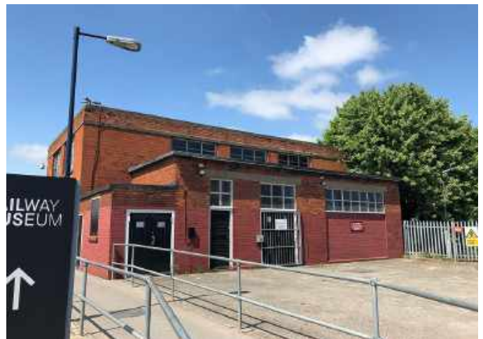
Fig.266 Generator building seen from the east
