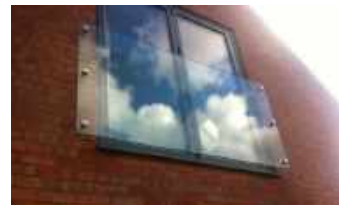
Glass balustrade to Juliette balconies ✗
