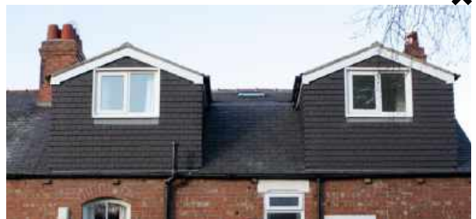
Fig.327 Not integrated with facade, dormer too big (dominates the roofline and elevation), windows too small, no articulation of dormer elevation, roof slope shows cheap roofing material, exposed gutter delivering to roof
