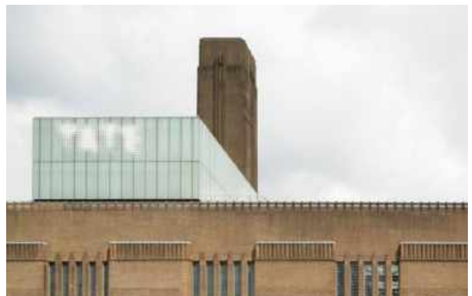
Fig.260 Example of a roof extension in material contrasting with the brick base
