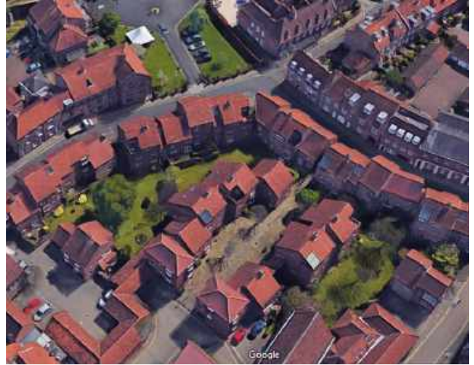
Fig.289 Small scale roofs to houses on St Andrewgate ✔️
