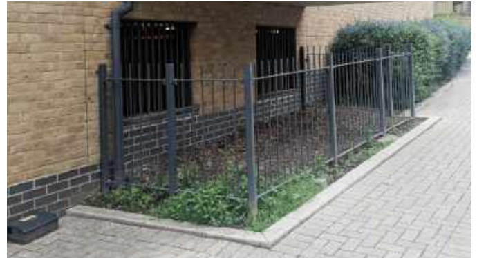
Fig.371 Barriers shall only be placed where required (note here the security grilles already over the windows)
